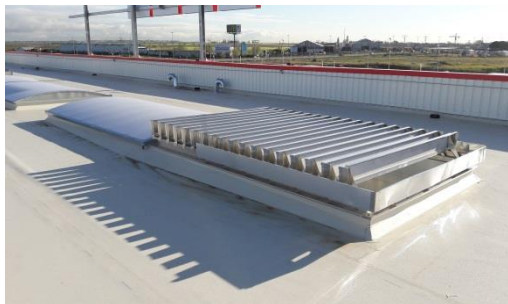
Auchan warehouses and shopping centres, Spain, smoke exhaust systems
