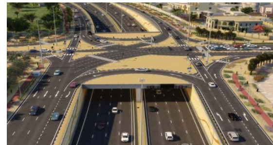
Al Rayyan Road Tunnel, Doha, Qatar, anti-fire construction protections
