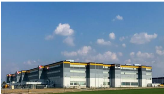
Amazon (Gliwice, Sosnowiec), Poland, fire ventilation and smoke exhaust systems
