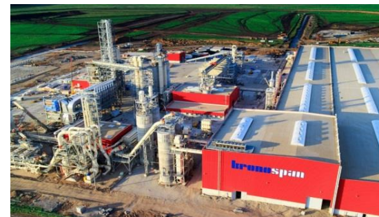
Kronospan plant, Russia, smoke exhaust systems
