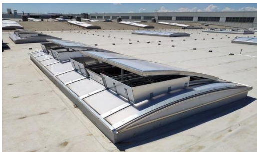
Faurecia plant, Hlohovec, Slovakia, smoke exhaust systems
