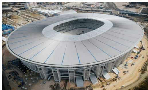
Puskás Aréna stadium, Budapest, Hungary, fire ventilation and smoke exhaust systems
